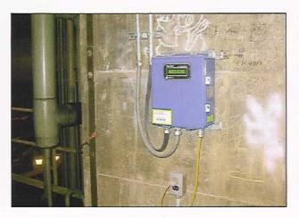
measure air in-leakage, water vapor flow, and up to eight additional performance parameters. The information can be used to troubleshoot condensers and vacuum systems and increase overall plant thermal efficiency.
