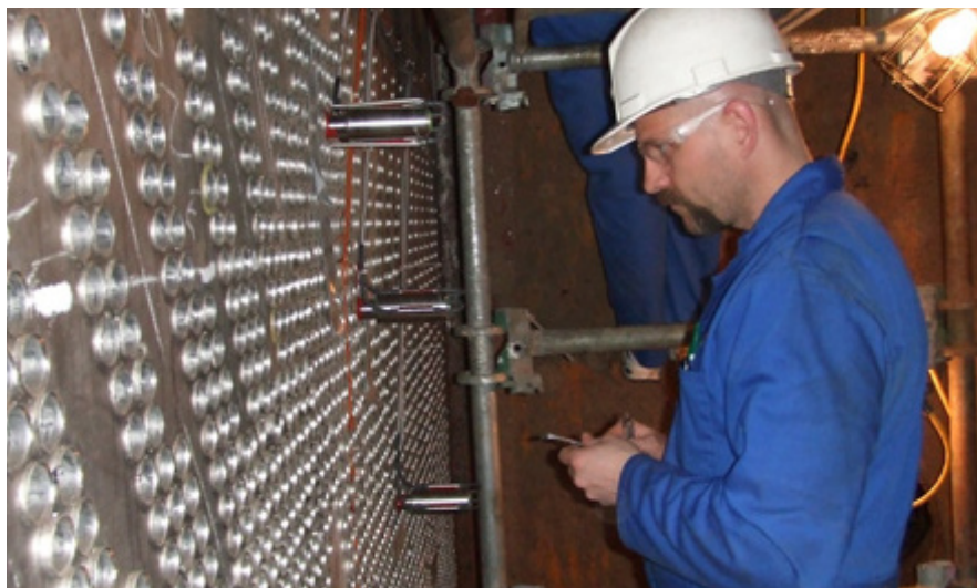
CWFF sensors installed on tube sheet. Waterbox compatible epoxy adhesive seals the units in place and protects signal transmission wiring.
